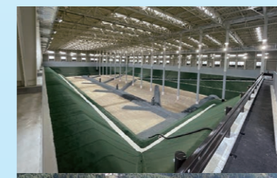
Kesennuma Disposal Site (2022) The forest in the Kujo district and surrounding areas was cleared to make way for this new final disposal site for municipal solid waste. The entire structure involved the following work: 195,040 m 3 of soil excavation and embankment, construction of a 410 m reversed T-type retaining wall, laying 23,792 m 2 of waterproof sheets, installing 321 m of groundwater collection pipes, installing 2,017 m of guttering, construction of a 4,014 m 2 concrete dam for the regulation pond used for disaster prevention, construction of a landfill gas treatment facility with five vertical pipes, and asphalt paving work for the 8,305 m 2 passageway. We also constructed a 9,760 m 2 storage facility covered with a roof (steel truss).
