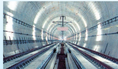
Seikan Tunnel (1982) This 53.8 km railway tunnel runs below the Tsugaru Strait, connecting Honshu (the Japanese mainland) and Hokkaido. Tobishima completed the 5.5 km Sanyoushi section on the Honshu side. Fraught with heavy technical challenges and constant flooding hazards, this project had significant consequences for integrating the nation and was selected as one of the 20 Selections of Japan's 20th Century Heritage.
