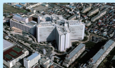
Kanagawa Science Park: KSP (1989) Developed by Kanagawa Prefecture, Kawasaki City, and TOBISHIMA, this collection of facilities serves as an international center where R&D companies are incubated and developed, gather, and interact, to formulate creative R&D movements. The project was recognized by various honors, including the BCS Special Prize and the Prize of the Society of Heating, Air-Conditioning, and Sanitary Engineers of Japan.
