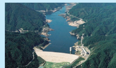
Surikamigawa Dam (2006) This rock-filled dam with a center core, one of the largest in the Tohoku region, supplies city water, including drinking water and water for other everyday uses to three cities and four towns, including Fukushima City. It also provides irrigation for rice paddies and agricultural land along the Surikami River and Abukuma River to support the thriving agriculture of this region.
