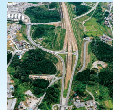
National Highway No. 45, Rikuzentakata Road (2018) This 10 km limited highway was planned as a leading earthquake disaster reconstruction project. We constructed the 7.0 km section on the side of Rikuzentakata. Completion of the road will strongly help afflicted areas move forward with local reconstruction and is expected to play a major role in the development of local industries encompassing Iwate and Miyagi prefectures.
