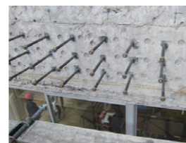
Blast key construction method
