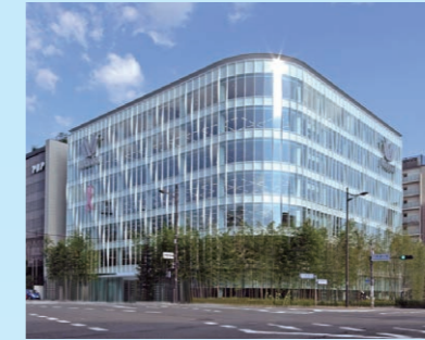
Wacoal New Kyoto Building (2016) Designed to serve as a new marketing base, the building with its external fins and other design features expresses tact, gentleness, refinement, and purity. Incorporating a toggle brace seismic damping structure, the building attained S rank class, signifying Superior quality by CASBEE.
