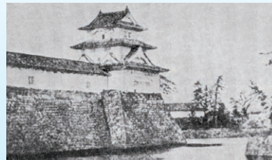
Demolition of Fukui Castle (1883) Bunjiro Tobishima founded Tobishima-gumi, which was contracted to demolish Fukui Castle as its first job.
