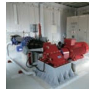
Water turbine generator (rated capacity: 136 kw)
