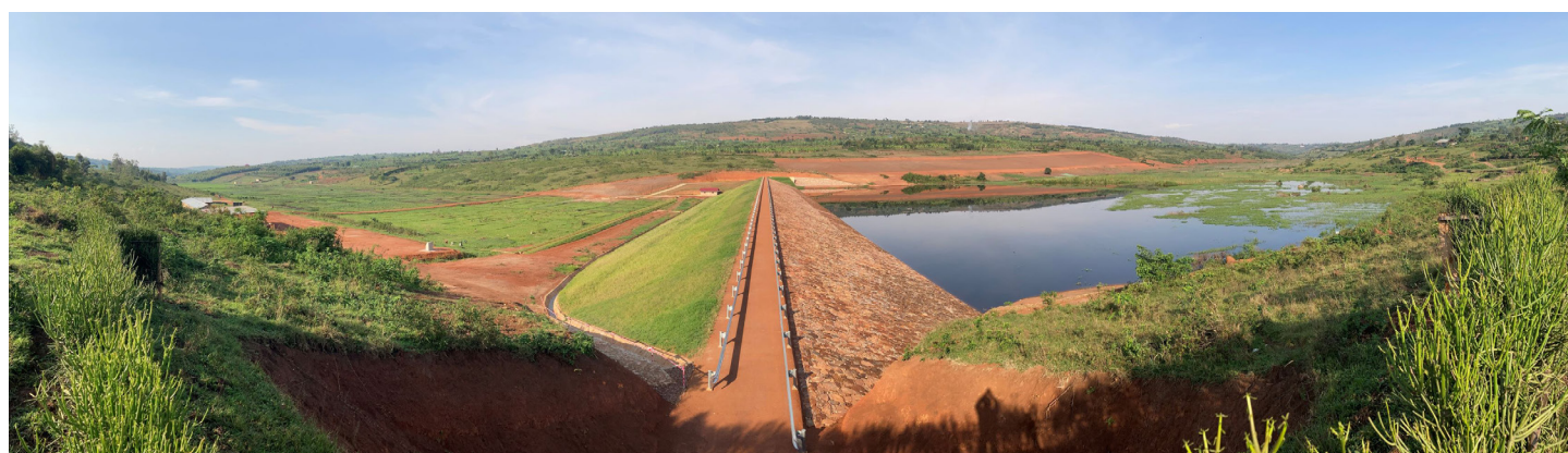
Rehabilitation of Irrigation Facilities in Rwamagana District [Rwanda]
