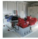
Water turbine generator (rated capacity: 136 kw)
