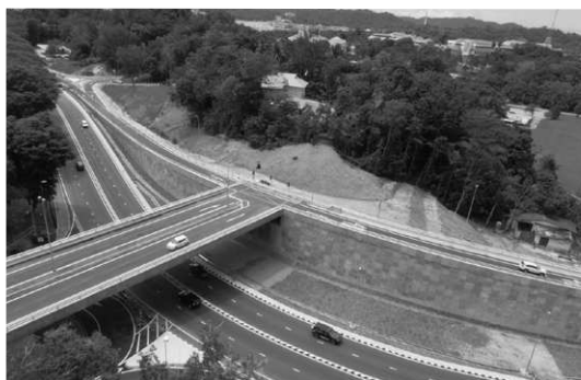
Construction of Interchange at Babu Raja -Tutong [Brunei]
