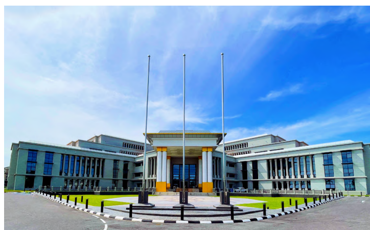
Brunei Darussalam Central Bank Building Project
