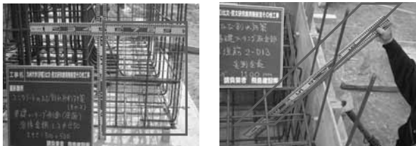
(1) 溶接金網φ3.2mm@50mm (2) 鉄筋D13,長さL=1100mm
