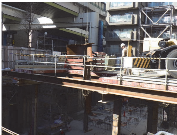
写真-4 構台下鉄骨建方状況
